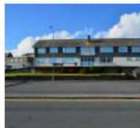
Public facilities out of date
