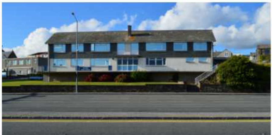
Public facilities out of date
